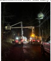
if necessary. Next, we would make repairs to the main distribution lines that directly serve a great number of homes and businesses. These overhead power lines are typically where we would begin with smaller outages caused by branches, animals, or vehicles. After those repairs are made, crews may work on tap lines which deliver power to transformers. Finally, individual service lines that run between the transformer and the home are repaired.
